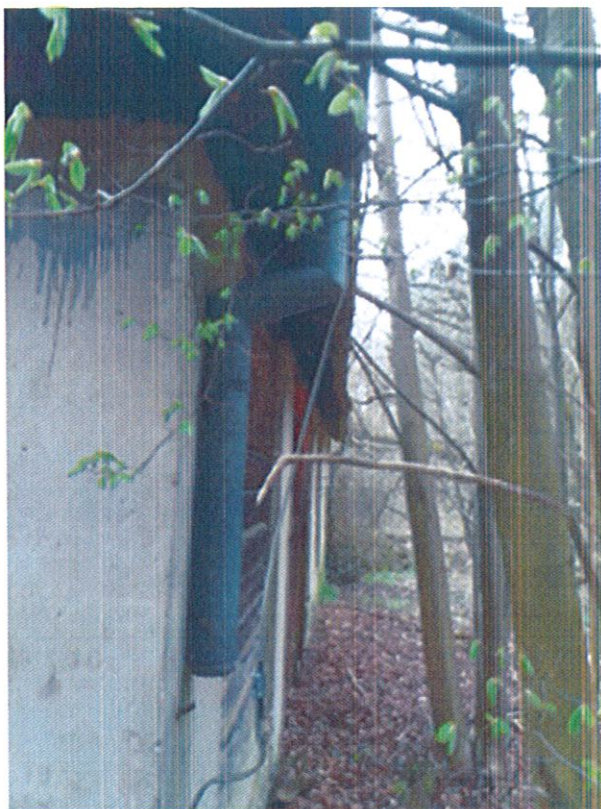
Oberwane rynny i rury spustowe
